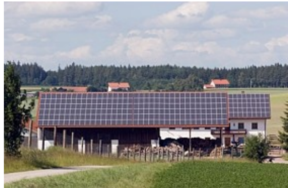
Solar Panels on a Farm Building
